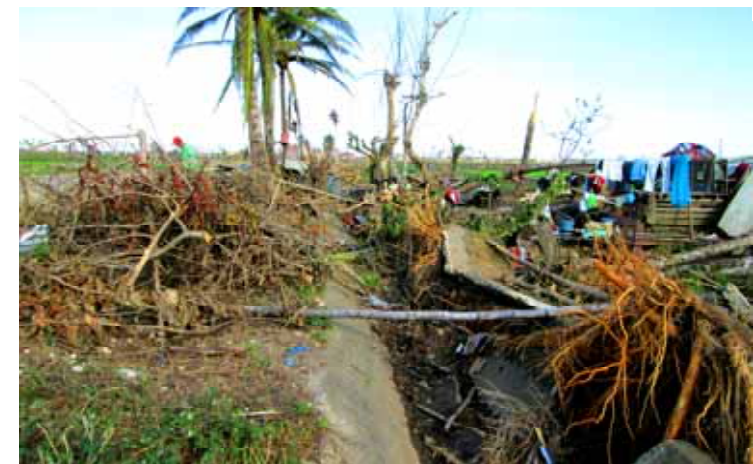
Destroyed canal at Abijod CIS, Cateel, Davao Oriental incurred during Typhoon Pablo's landfall on December 4, 2012.
